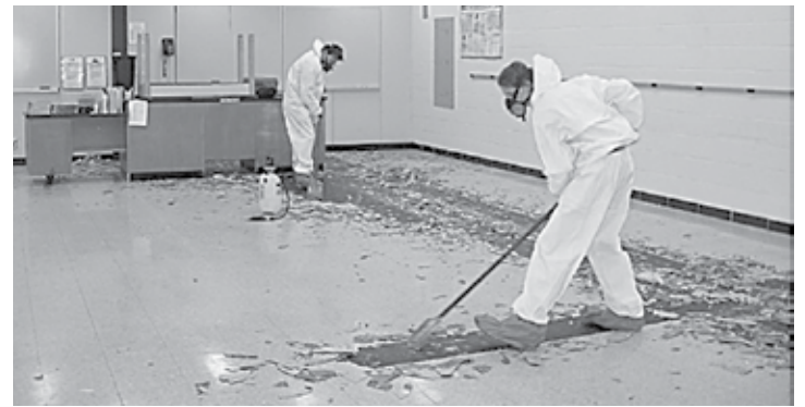
Asbestos-containing floor being removed from a JHS classroom as part of the renovation plan.
